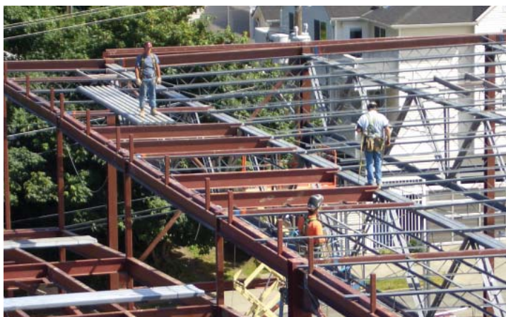
July 2006: The steel structure of the new commons/gymnasium is in place.
