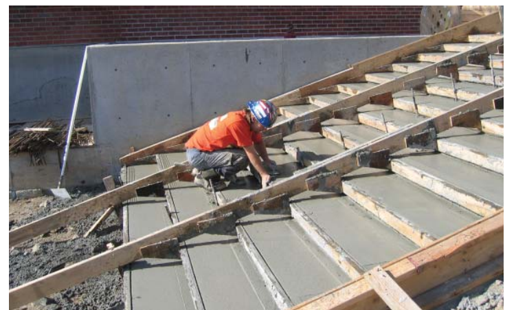
June 2007: Concrete for the grand stair is poured at the east entry.
